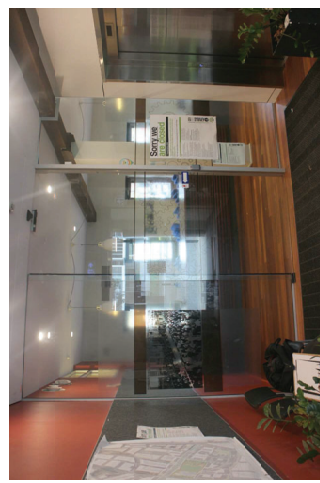
FIG 1 EXIST TENANCY GLASS ENTRY, AUTO SLIDE
