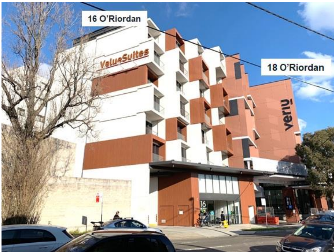
Figure 13: Hotel developments at 16 and 18 O'Riordan Street adjacent to the south.
