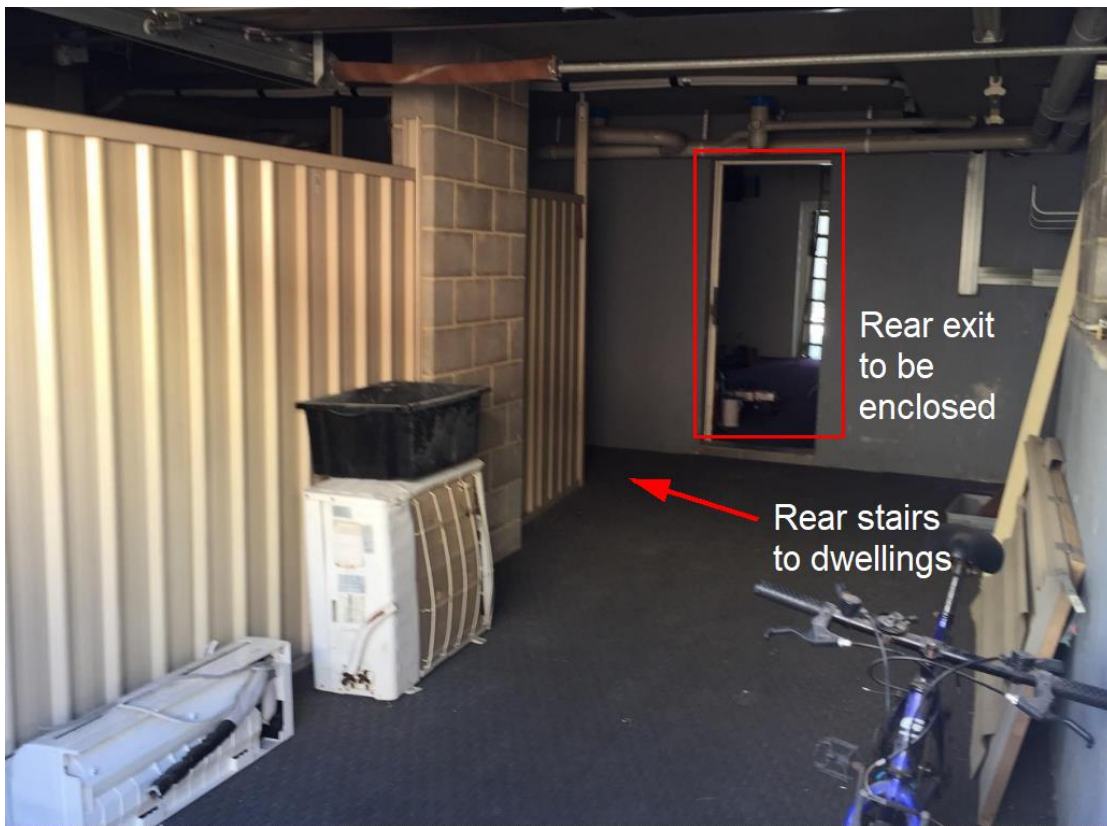
Figure 4: Rear access adjoining proposed staff room and adjoining residential garages
