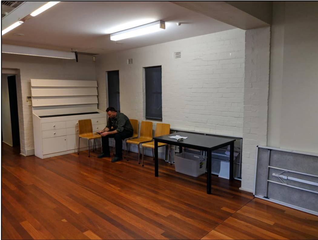
Figure 8: Existing painted brick walls and timber framing will be retained. Modern cabinetry and skirting containing wires will be removed.
