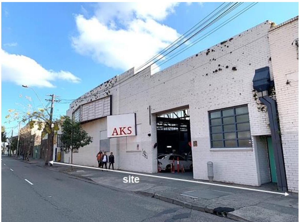
Figure 2: Botany Road frontage of subject site.
