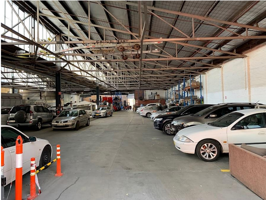
Figure 9: Interior of existing warehouse looking west.
